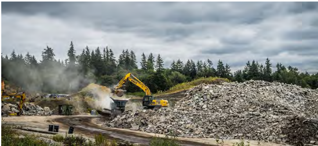
Figure 17. Current Mining Activities on Milton's Quarry Site
