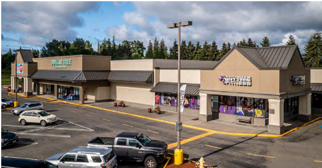
Figure 8. Commercial Buildings on Meridian Avenue
