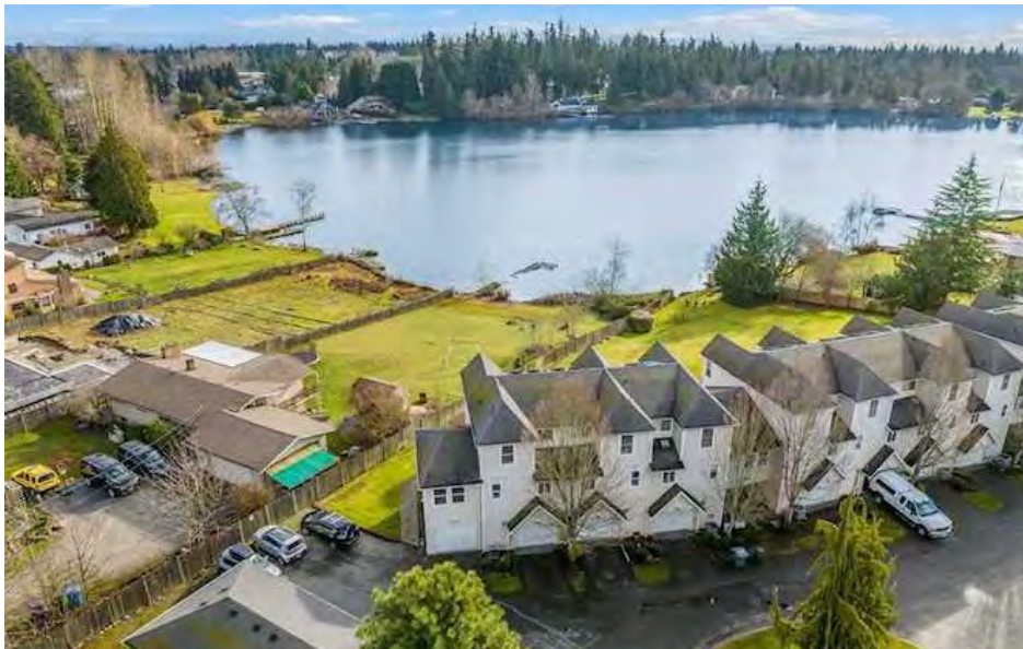
Figure 41. Lakeside Residential Development
